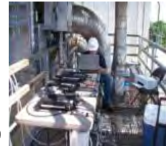
Multi-point NO x /O 2 Analyzer Set-up
